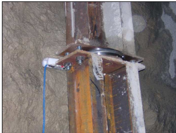
LOAD CELL MOUNTED BETWEEN STEEL SUPPORT SEGMENTS
